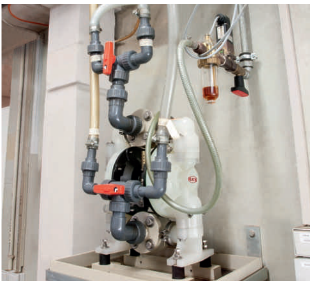
FDM: Pumping of chemical nickel for electroplating bath.
